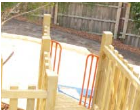
This has good handrail definition, but the bright background surface might be difficult
