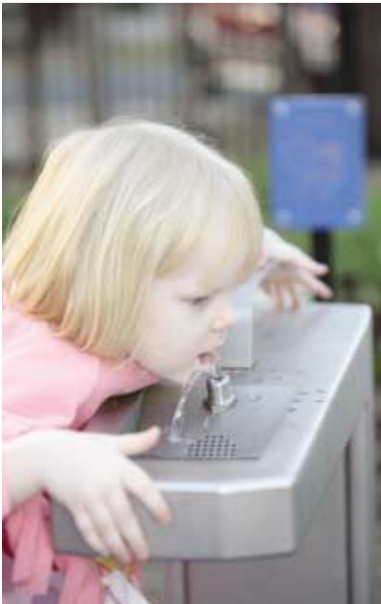
Drink fountains need to be able to be reached, without wetting a person in a wheelchair. They should be able to fill a cup or drink bottle and have levers that are easy to operate
